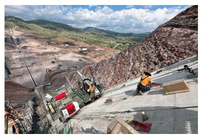
Grouting on the east abutment at Chimney Hollow Reservoir took place on 45degree angles.
