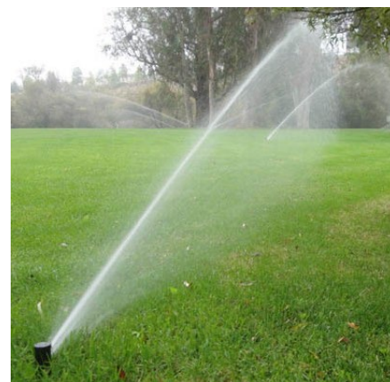
Rotors broadcast irrigate large open turf or native seed landscapes
