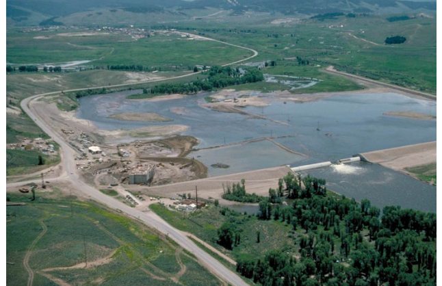
Construction of Windy Gap Reservoir.
