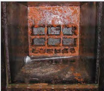
Corrosion on the left guard gate
