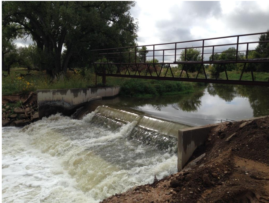
Figure 4. Newly Installed Beeman Ditch Diversion Structure Using Obermeyer Crest Gates on South Platte near Platteville With Gates in Up Position
