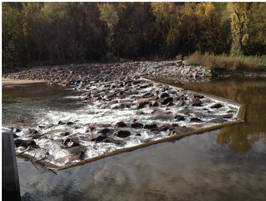
Figure 2. Rough and Ready Grouted Boulder Diversion Dam Structure
