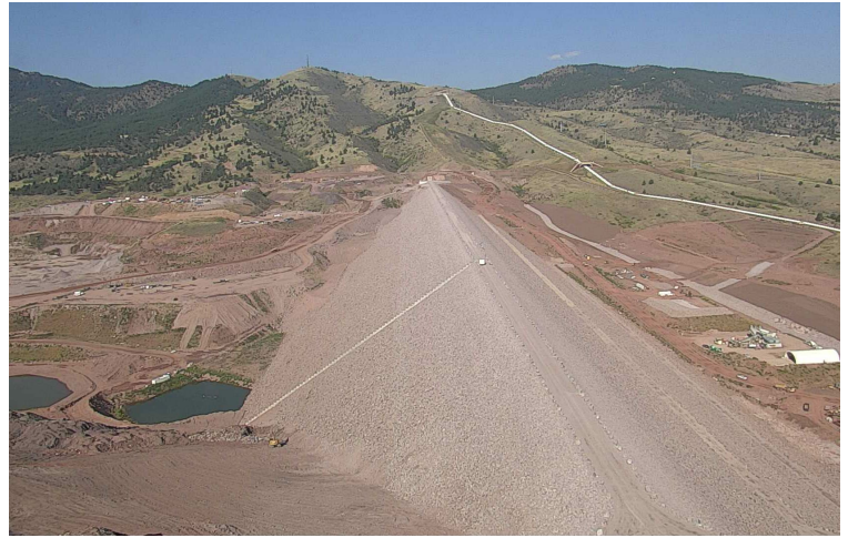
Construction of Chimney Hollow Reservoir was complete in late 2025.
