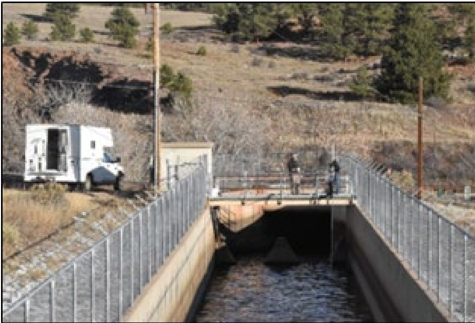
Figure 4 – Water quality sample collection on the Hansen Feeder Canal.
