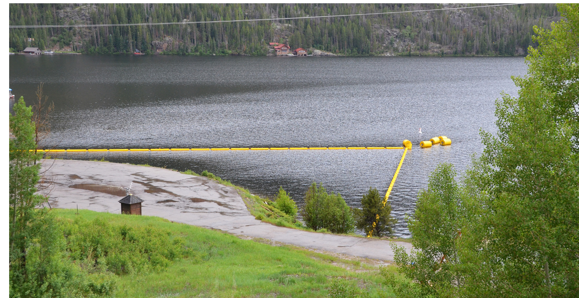
Debris Boom at West Portal
