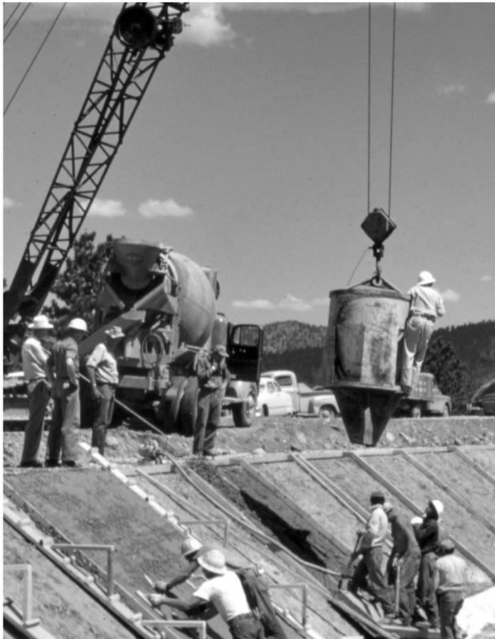
Crews work on installing concrete panels for the Pole Hill Canal in 1952.
