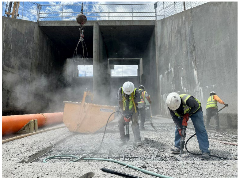
Improvements were made at the Shadow Mountain Reservoir spillway in 2025.
