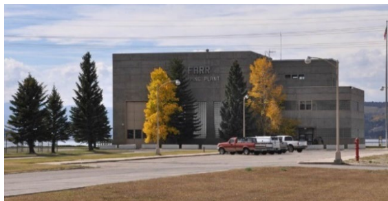
Farr Pump Plant
