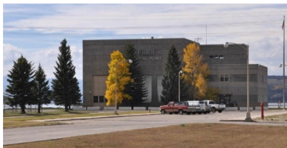
Farr Pump Plant
