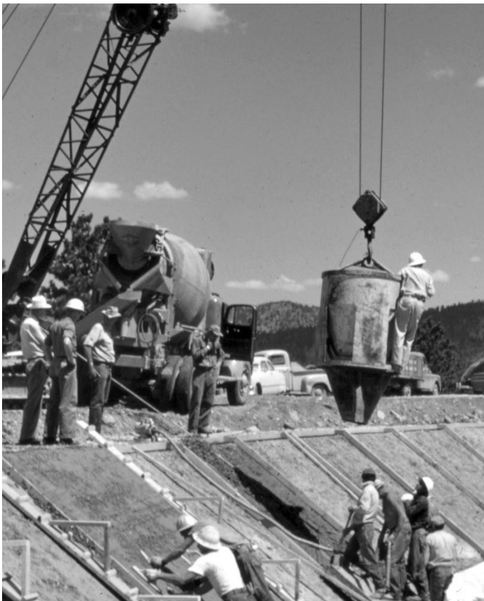
Concrete panels are being constructed for the Pole Hill Canal in 1952.
