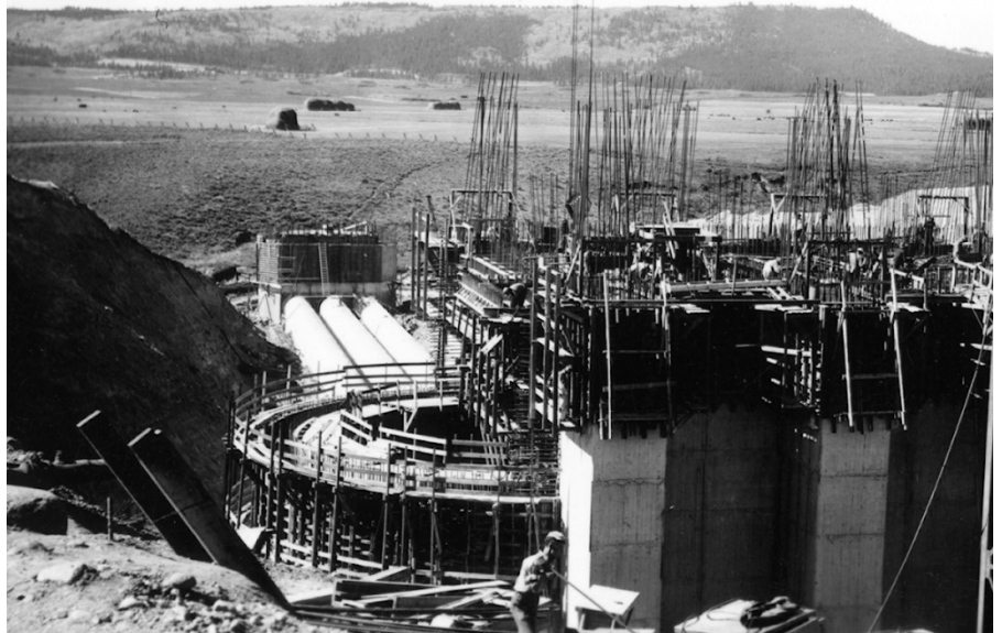
Crews construct the inlet structure on the Granby Pump Plant, later renamed Farr Pump Plant, in September 1948.
