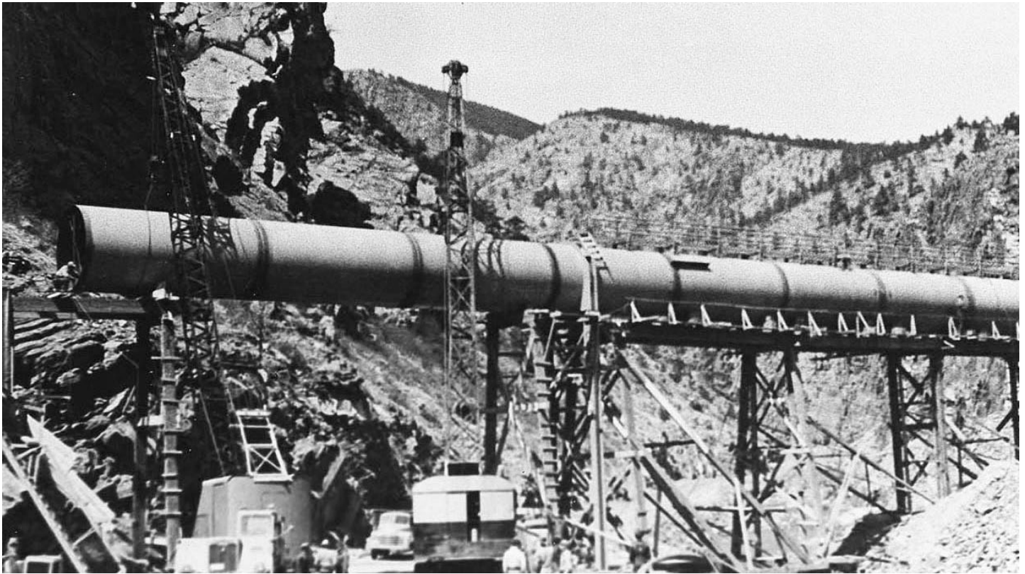
Crews constructing the Big Thompson Siphon at the mouth of the Highway 34 canyon toward Estes Park.
