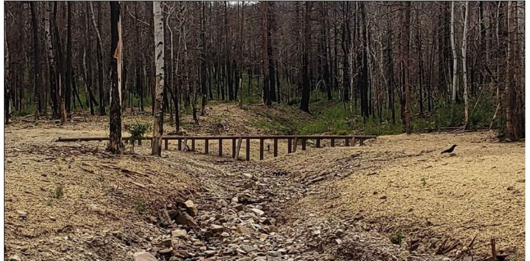
Steel debris barrier before flood (TJ Burr, NRCS, 6/25/2020)
