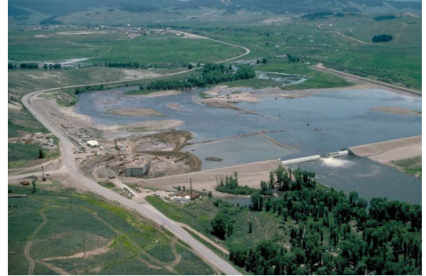
Construction of Windy Gap Reservoir.
